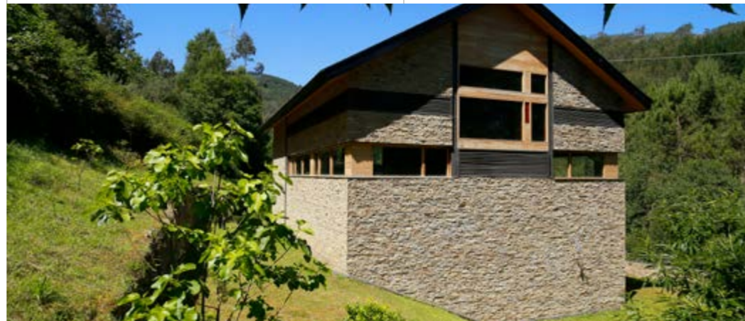
Landro hydroelectric power plant (Ouro, Lugo, Galicia).
