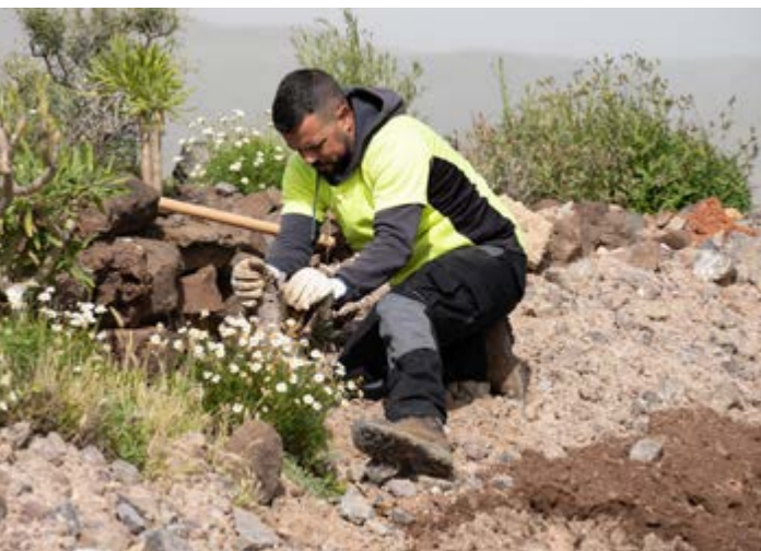
Revegetation process in the wind farms of La Gomera.
