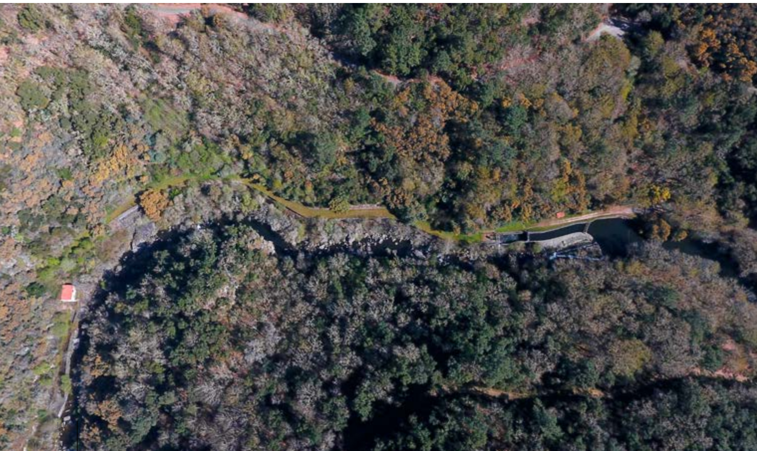
View from above of the water intake of the Arnoya hydroelectric power plant (Ourense, Galicia, Spain).
