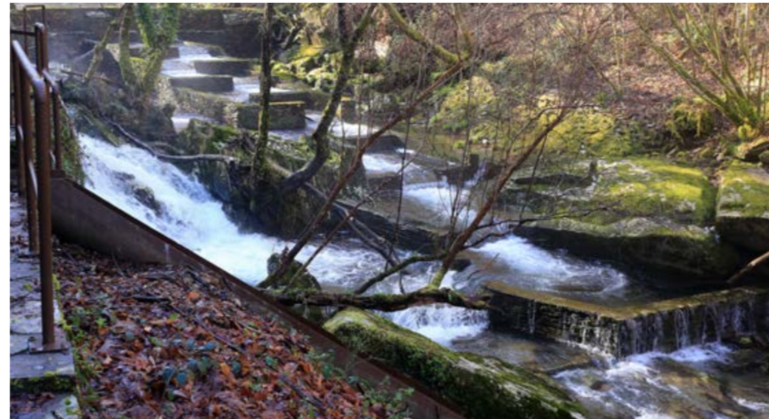
Fish ladder from water reuse at the San Bartolomé hydroelectric power plant (Galicia, Spain).
