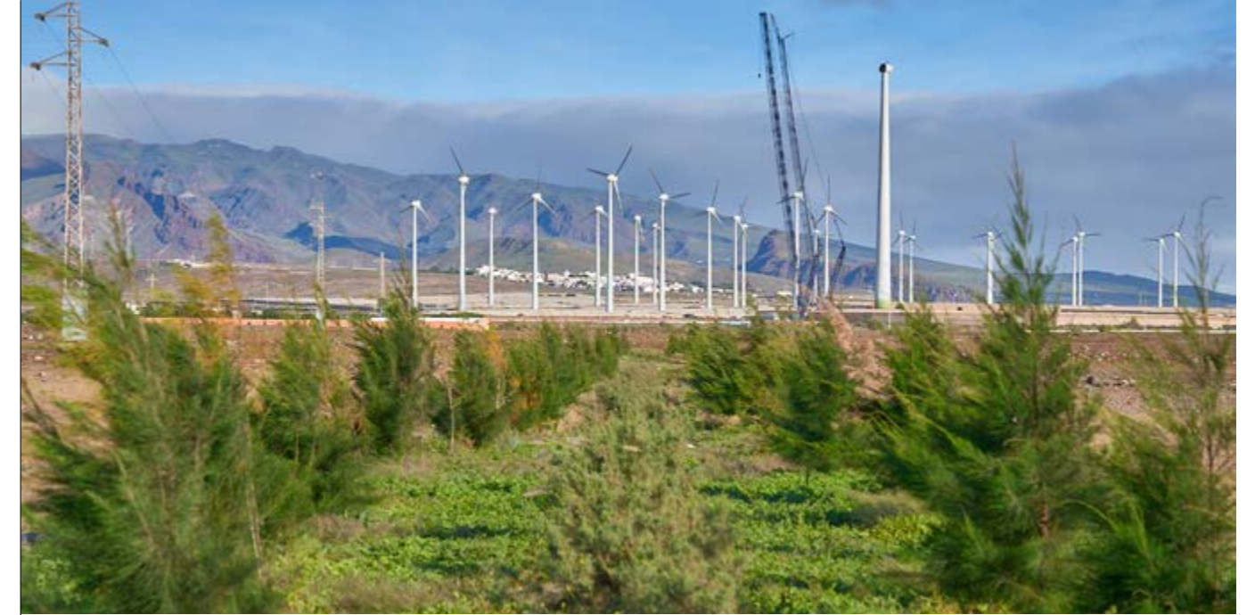
Vegetation screen planting process, an environmental measure carried out at our facilities in the Canary Islands.
