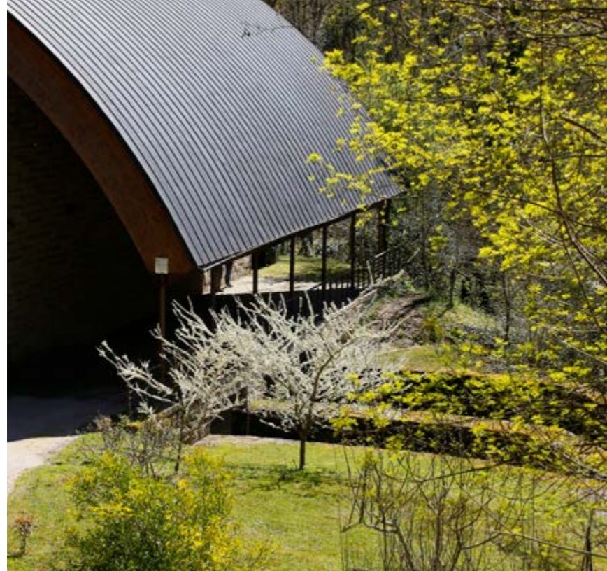
Peneda hydroelectric power plant (Ourense, Galicia, Spain).
