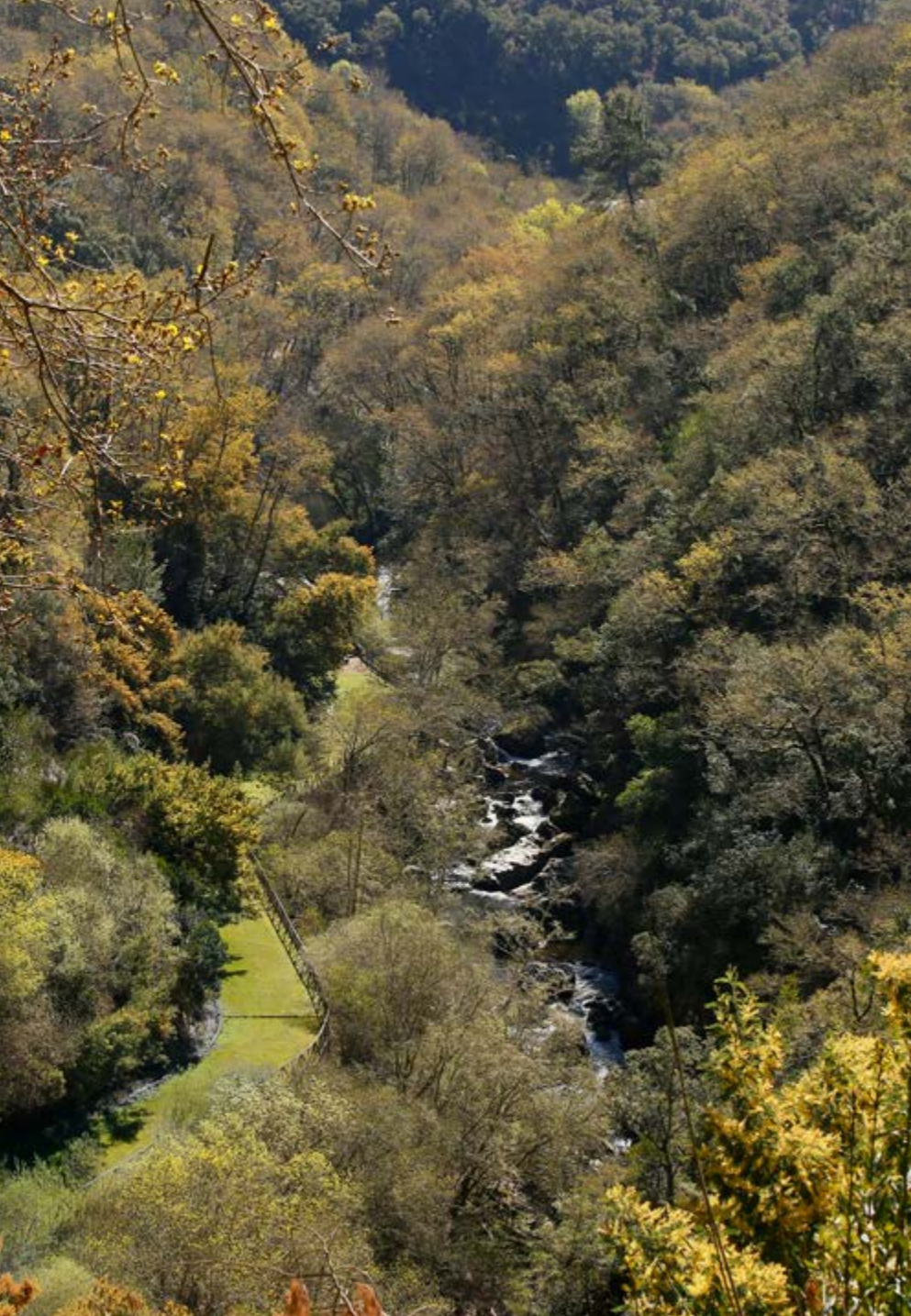
Buried bypass channel; the photo shows a green space for walking. It belongs to the Arnoya hydroelectric power plant (Ourense, Galicia, Spain).
