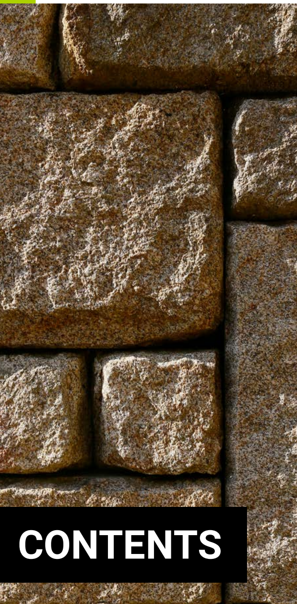
Close up image of the Ciervas hydroelectric power plant (Galicia, Spain) built from granite.
