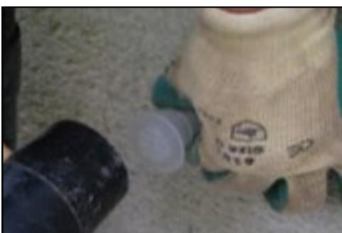
**Note:** Spacing of drill vents for ventilation or drainage may vary depending on the specification, Building Regulation requirements, building type or location.
