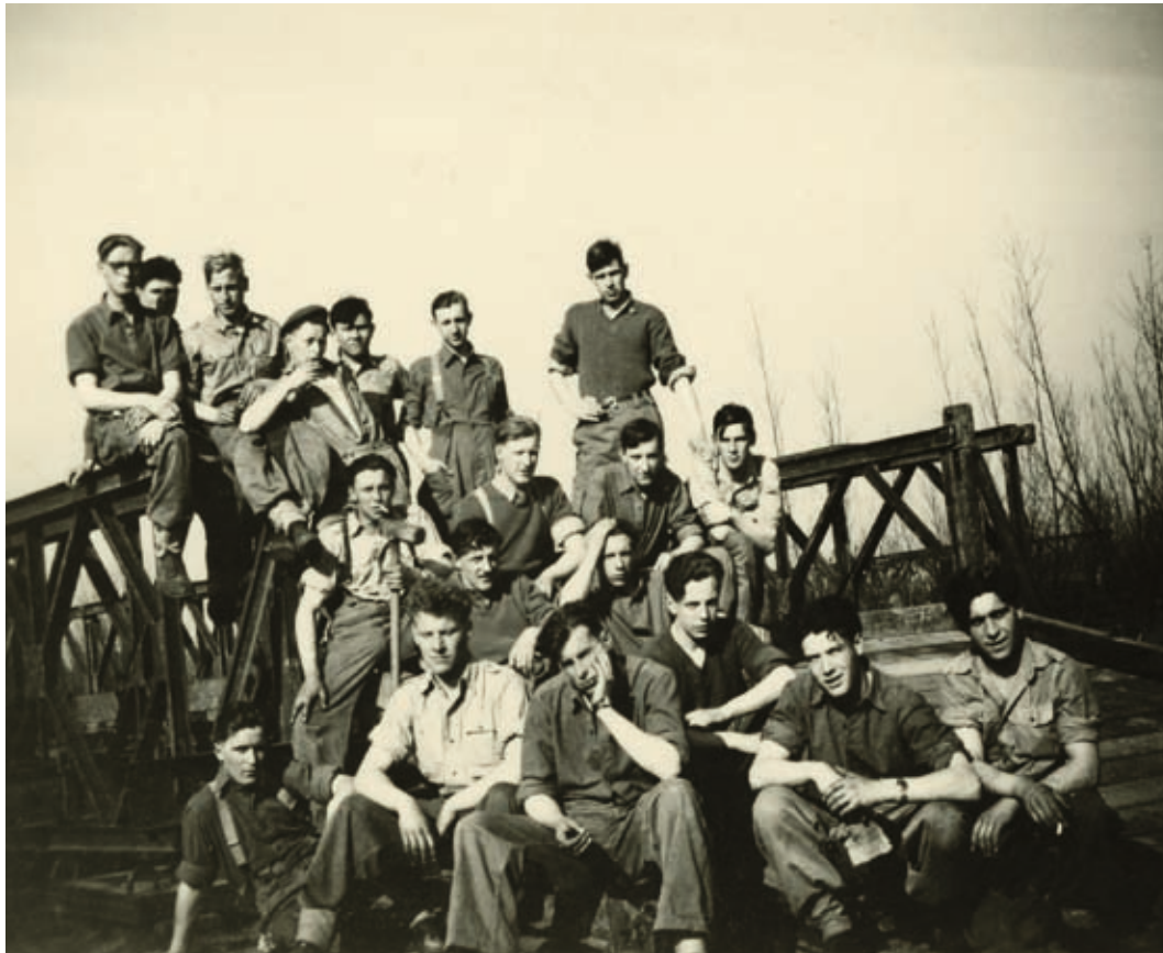
3RD PELOTON PONTONNIERS CONSTRUCTING A BAILEY BRIDGE ACROSS THE RIVER MAAS AT WELL LIMBURG IN 1953.
