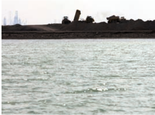
Trucks dumping soil onto site to build up land from barges
