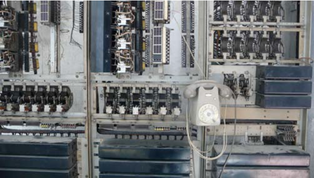
TANTALUM MEMORIAL – RESIDUE, 2008 1938 TELEPHONE EXCHANGE CONNECTED TO SOCIAL TELEPHONY NETWORK
